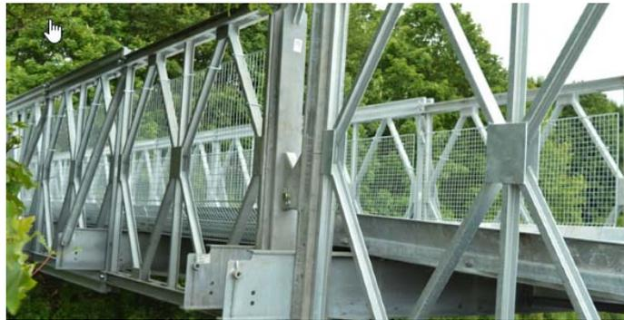
**Figure 19:** Modular Bridge Protective Screen System
