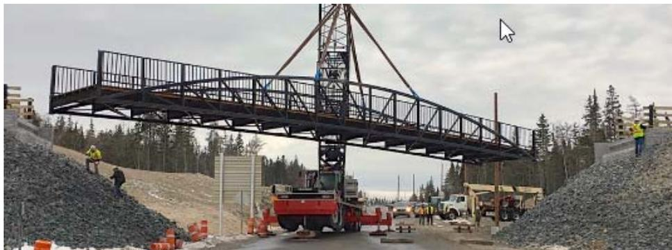
**Figure 6:** Installation of a Bowstring Truss Bridge
