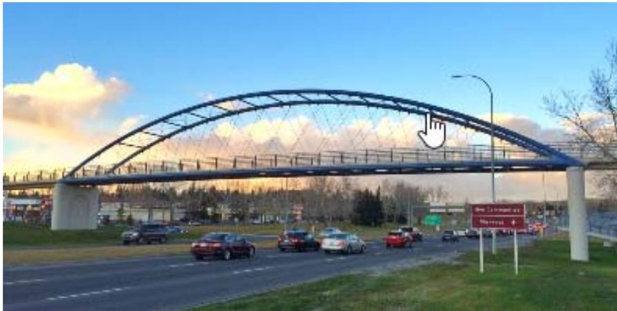
**Figure 10:** Network Arch Pedestrian Bridge Example
